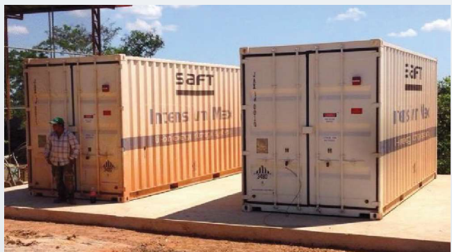
Saft Intensium® Max at Cobija, northern Bolivia - the world's largest hybrid PV-diesel microgrid
