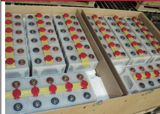
Batteries are placed in an upright position with polystyrene filling out the crate so that no movement can take place.
